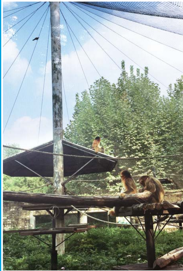
Monkey cage enclosure, 3600 m 2 Chengdu Zoo Zoomesh wire rope dia.: 2.0mm Zoomesh aperture: 51mm x 51mm
